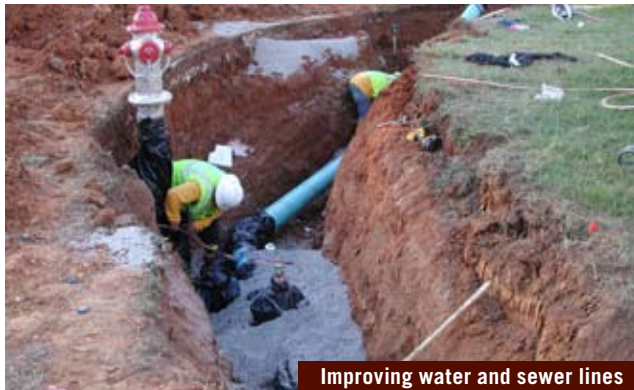
Improving water and sewer lines
